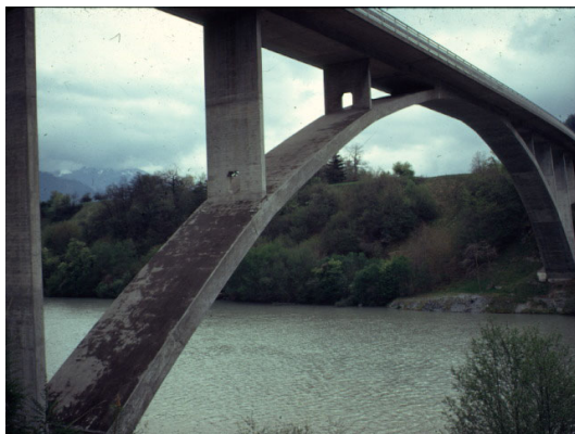
Figure 17 – Wide Spacing Between Crosswalls (Photo by D. P. Billington)
