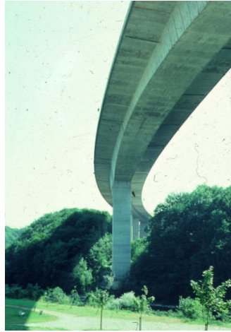
Figure 4 – Curved Box Girder (Photo by D. P. Billington)
