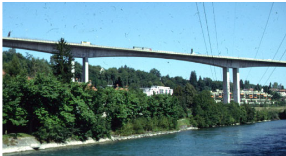
Figure 1 – Felsenau Bridge (Photo by D. P. Billington)
