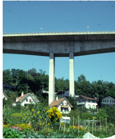
Figure 5 – Two-wall Pier (Photo by D. P. Billington)
