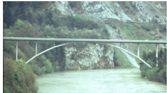
Figure 2 – Reichenau Bridge (Photo by Christian Menn)
