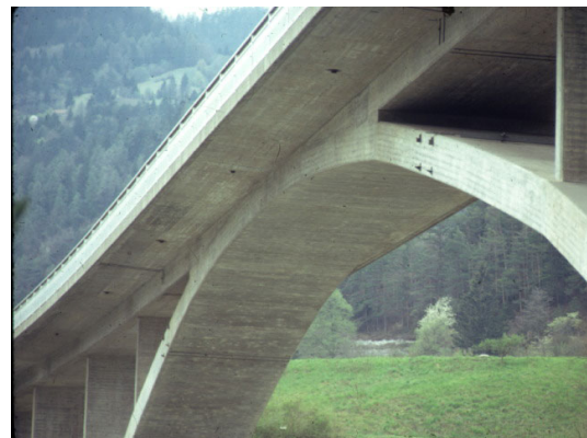
Figure 18 – Overhang of Deck (Photo by D. P. Billington)
