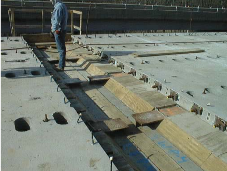
Fig. 2 Full-Depth Deck Panels on the Route 29 over Sugar Creek Bridge in Illinois
