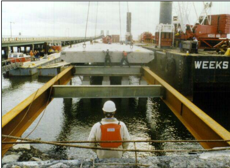
Fig.3 “Quad-Tee” Superstructure Units on the Robert Moses Causeway in New York
