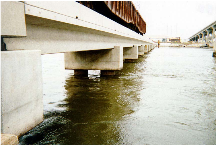
Photo courtesy of the North Carolina Department of Transportation
