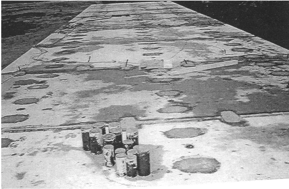
Figure 10. Deck with all Joints and Pockets Filled
