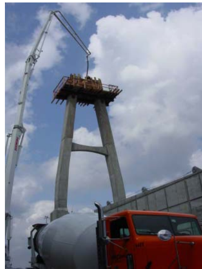
Fig. 12 East side pylon placement
