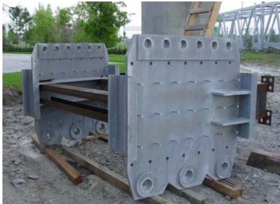
Fig. 2 Embed for top of 90 ft. high pylon
