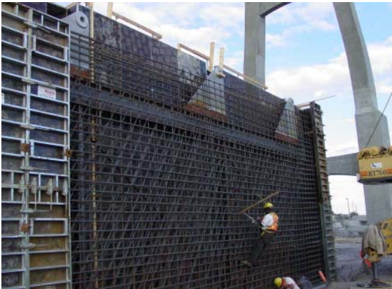
Fig. 1 Cable anchor wall with 10 ton embed
