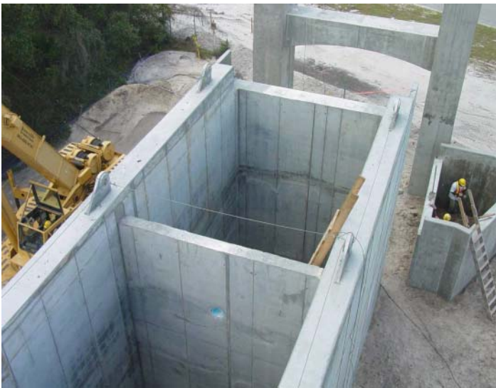
Fig. 11 Completed west side cable stay anchor
