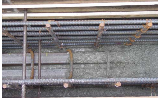
Fig. 10 S.C.C. easily encapsulated the embeds
