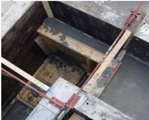
Fig. 9 Two foot high steps at top level
