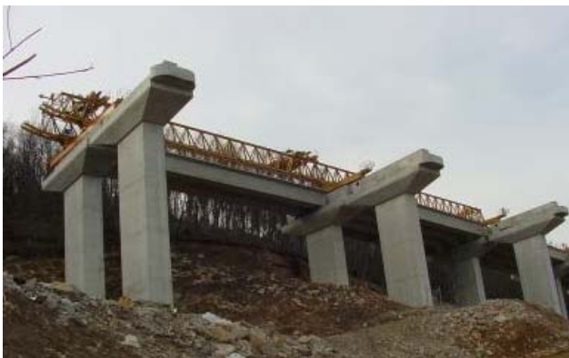
Figure 8: Girder launching
