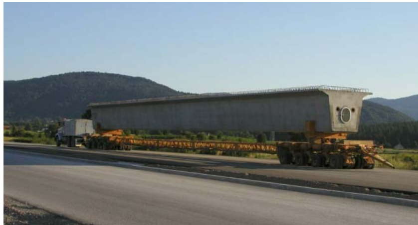
Figure 5: Girder transport on Capperi trailer
