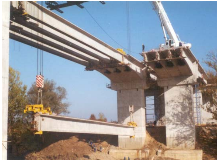
Figure 7: Girder placing at Kupa River crossing - Viaduct Dreznik
