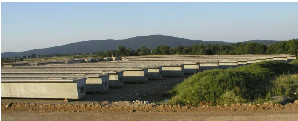
Figure 6: Girder storage at site
