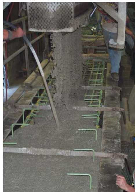
Fig. 4 Production of T Girders
