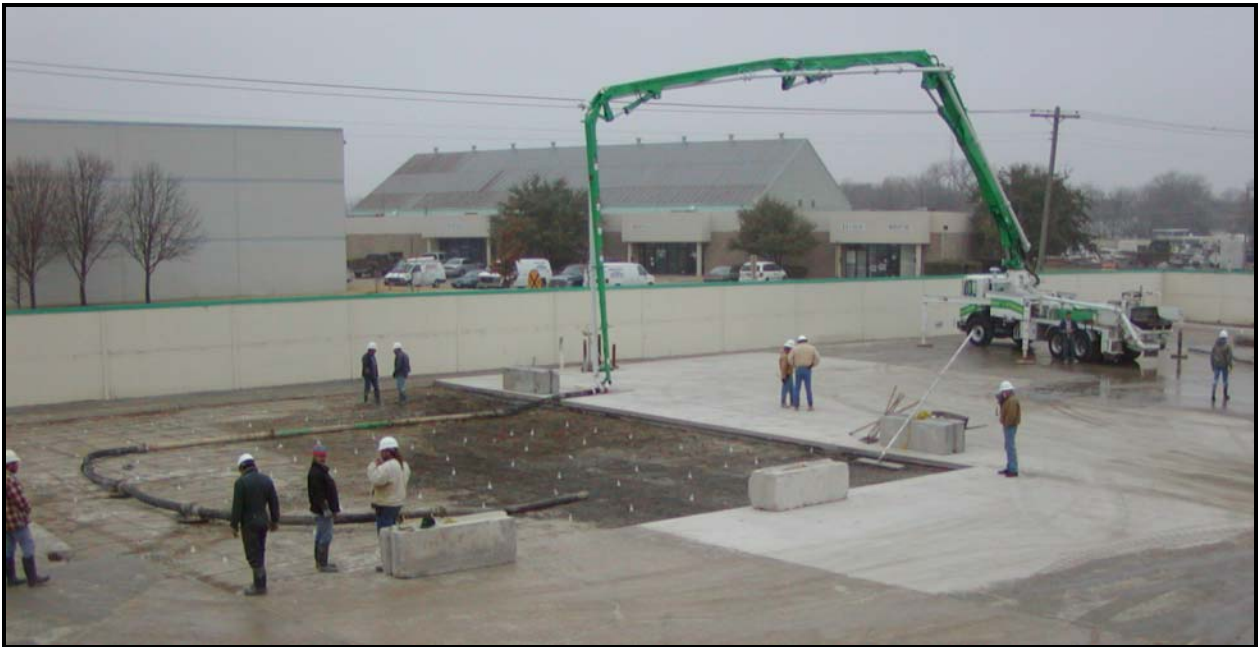
Fig. 6. Phase II pumpability testing
