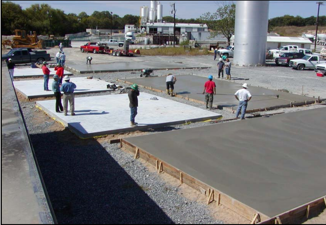
Fig. 1. Photo of tests slabs for Phase III
