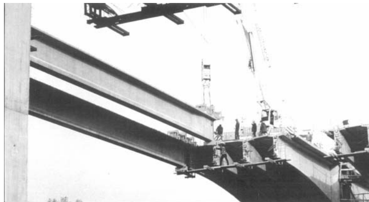
Fig. 8: Girder erection from river
