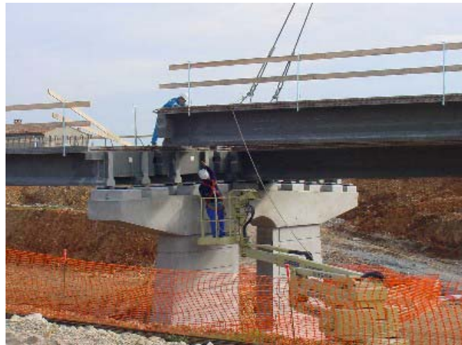
Photo 12 – Erection of a precast beam
