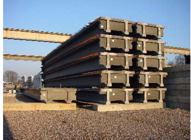
Photo 11 – Temporary storage of beams
