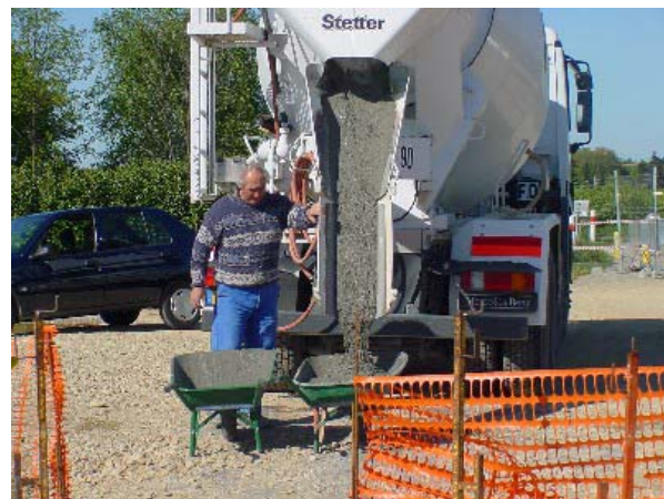
Photo 14 – BSI placed in wheelbarrows
