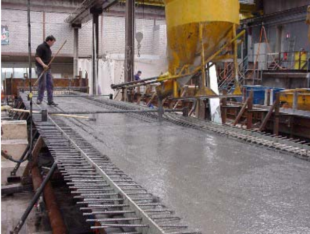
Photo 10 – Flange concrete placement
