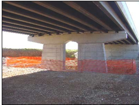
Photo 15 – View of completed bridge
