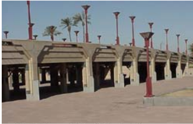
Central Avenue Viaduct, Phoenix, Arizona
