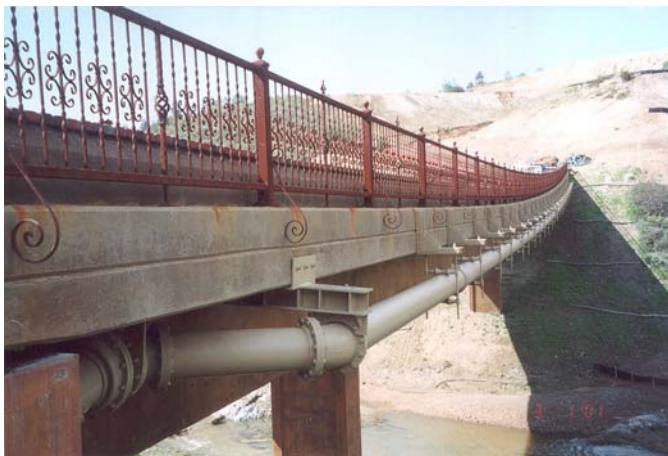
Vista Canon Bridge, San Diego County
