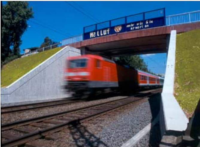
A railway overpass in Walluf, Germany.
