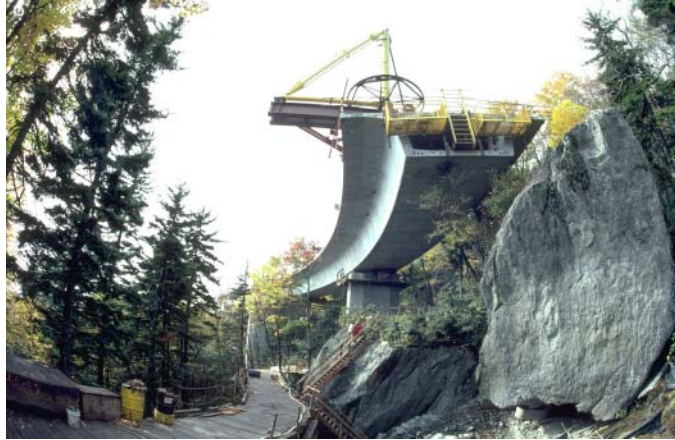
Black iron oxide was randomly mixed into the concrete used to build the Linn Cove Viaduct, to match the rocks of Grandfather Mountain.
