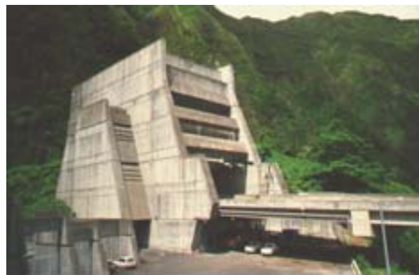
Portal to tunnel on Highway 3 in Hawaii
