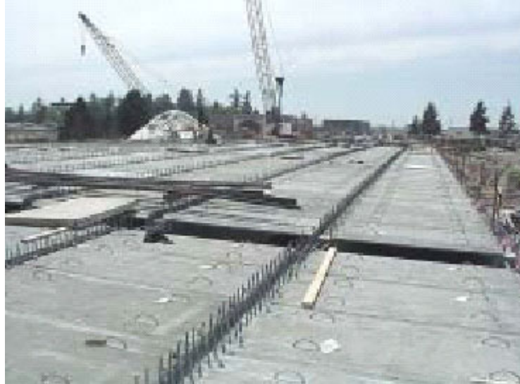
Fig. 1 Partial-depth precast concrete deck panels on I-5 Interchange in Tacoma, Washington
