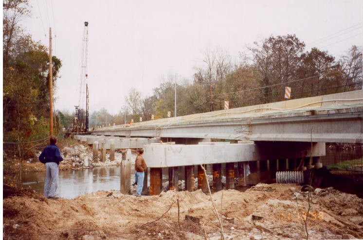
Fig. 4 Precast bent caps on Route 5 Bridge over Wolf River in Tennessee
