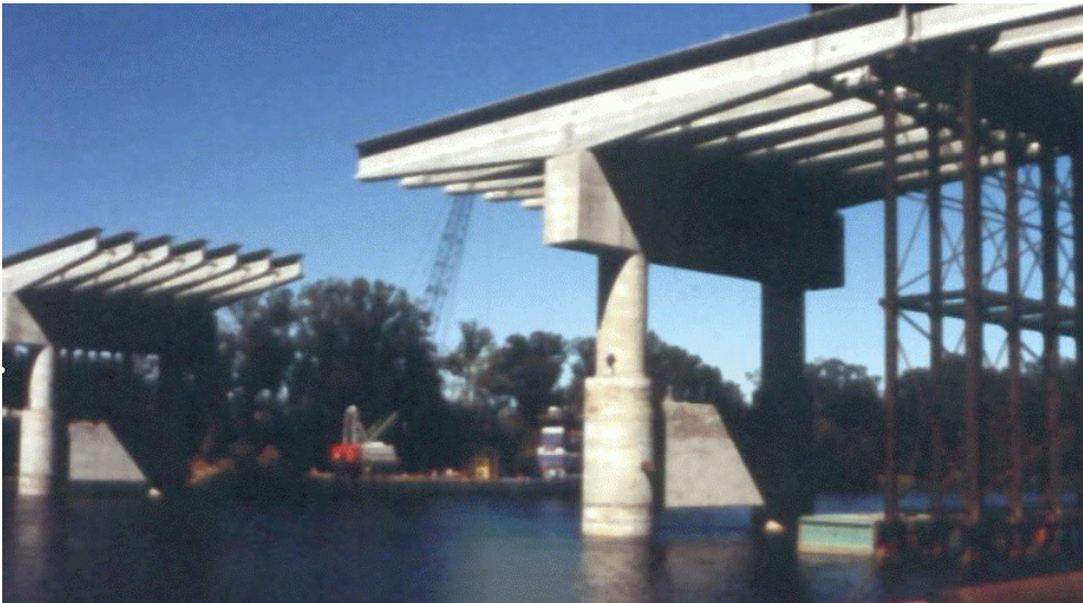
FIGURE 8 Black Warrior Parkway, An Example of a Spliced-Girder Bridge
