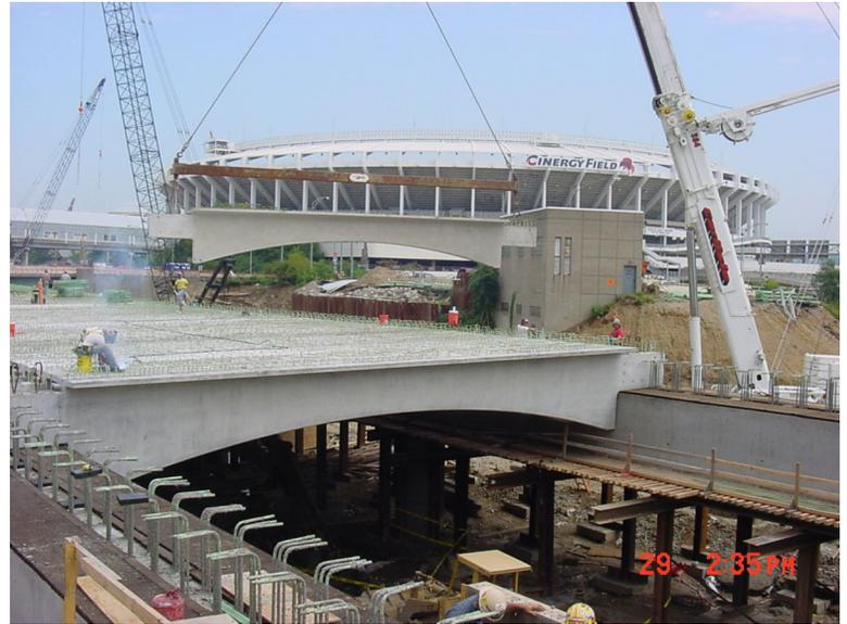
*Fig. 11 - Floor beam erection*
