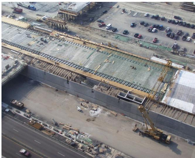
*Fig. 12 – Floorbeams erected awaiting deck slab castina*
