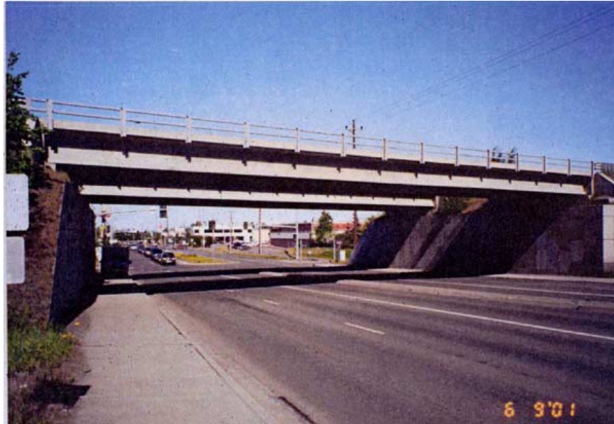
Fig. 5 Huffman Road Bridges, Anchorage, Alaska
