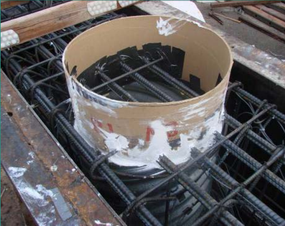
Sonotube Dam at Cap Top
