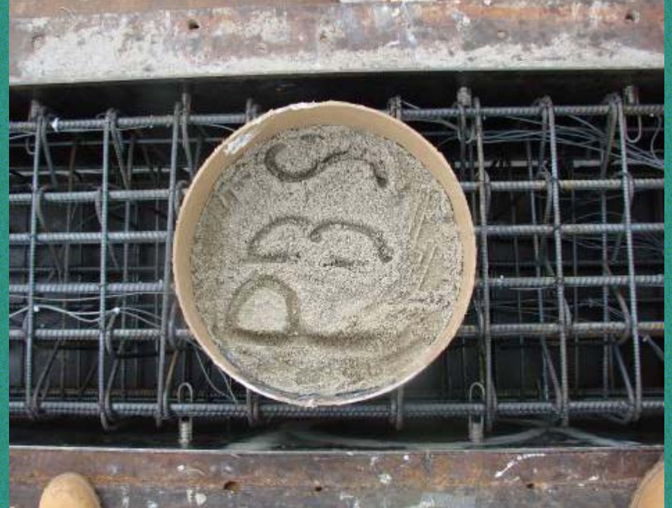
Sand in Sonotube Dam At Cap Top
