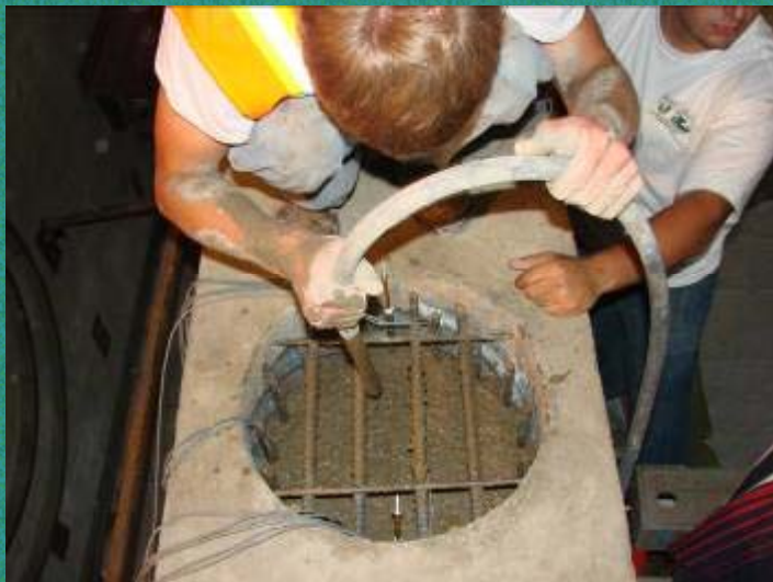
Casting and Vibrating Concrete
