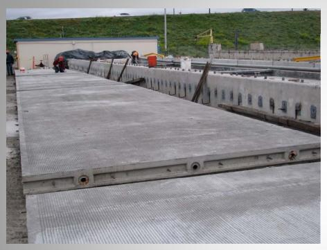
Cutaways in keyways for post Tension ducts, allows for alignment Recessed pocket for gasket minimizes grout leakage
