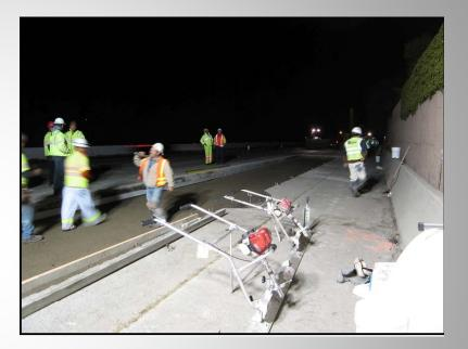
• Use gang drill to ensure longitudinal alignment when dowels are inserted.
