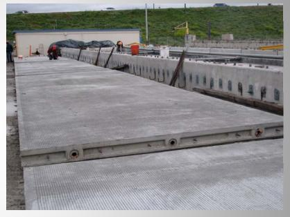
• 3 post-tension ducts (2" diameter), unlike original FHWA design (6 ducts).
