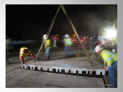
• After last panel is placed, remove temporary strands and perform final post tension on epoxy coated strands (5600 psi).
