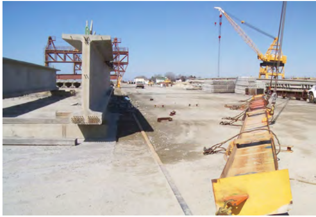
CRANE BRAKE FAILED AND DROPPED SPREADER BEAM ON GIRDER
