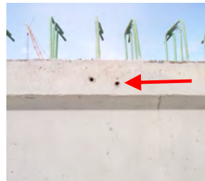
MISALIGNMENT OF INSERTS – OUT OF TOLERANCE
