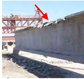
CRANE BRAKE FAILED AND DROPPED SPREADER BEAM ON GIRDER
