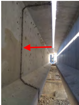
FORM OFFSET OUT OF TOLERANCE
