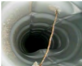
COLLAPSED AND PUNCTURED PT DUCT IN SPLICED GIRDER
