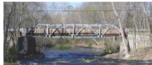
The existing bridge had met its life expectancy. Photo: Ralph Sweet.
