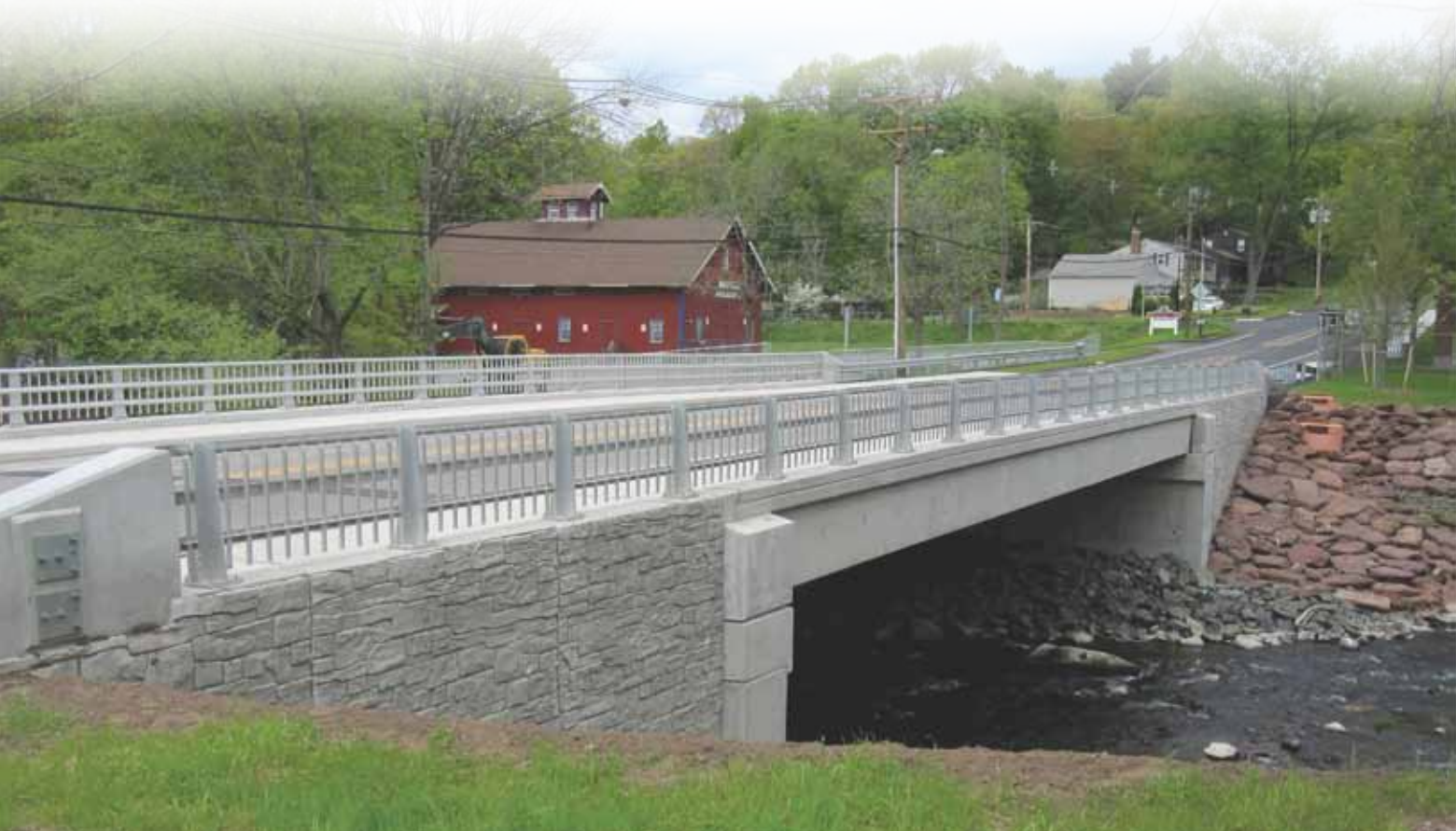
The handsome new South Maple Street Bridge features an ashlar stone texture cast on the wingwalls. Photo: Hoyle, Tanner & Associates Inc.
