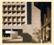
Fig. 11 – Deep recessed windows and overhang (eggcrate device). Photo: @ MBA
