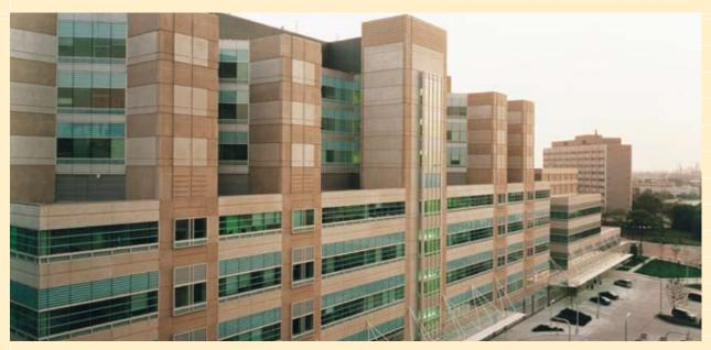
Fig. 36 – Insulated sandwich wall panels. John H. Stroger, Jr. Hospital of Cook County, Chicago, IL CCH Design Group headed by Loebl Schlossman & Hackl Photo: @Hedrich Blessing
