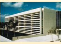
Fig. 5 – Freestanding screen. modest projections can be equally effective in shading but they must be more closely spaced. Closely spaced horizontal or vertical planes may begin to dominate the view out of a window and in any case change the scale of the window. The proportion of the space divided by the shading planes becomes as important as the overall window proportion in determining the aesthetic effect of the fenestration.
