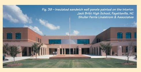
directly from the supporting footing. This is very important in reducing heat losses to the ground, especially where deep frost lines prevail. Also, by allowing the roof connection to be contained on the interior layer only, sandwich panels can provide a continuous insulation envelope, even at the roof-to-panel connection.
