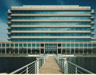
Fig. 2 – Horizontal sunscreen. Photo: @ Brian Gassel/TVS & Assoc.
