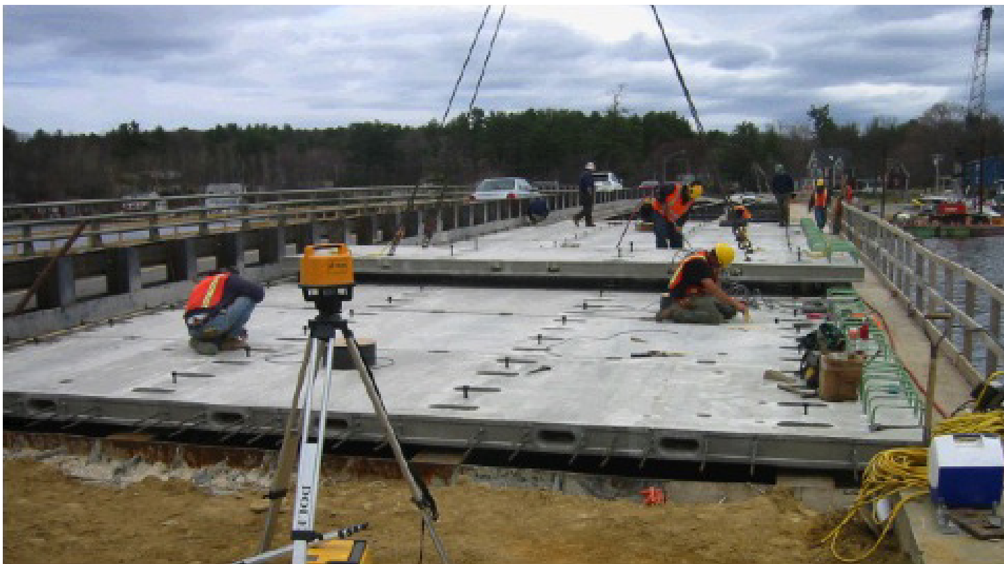
Figure 3.3.2-1 Placing Deck Panels
