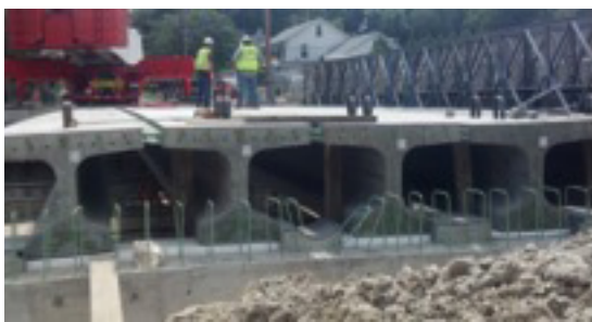
Figure 3.3.1.2-1 Deck Bulb Tee Construction
