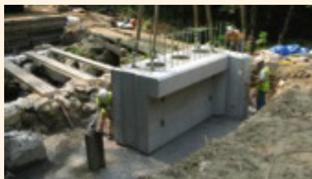
Figure 4.4.3-1 Precast Integral Abutment Construction
