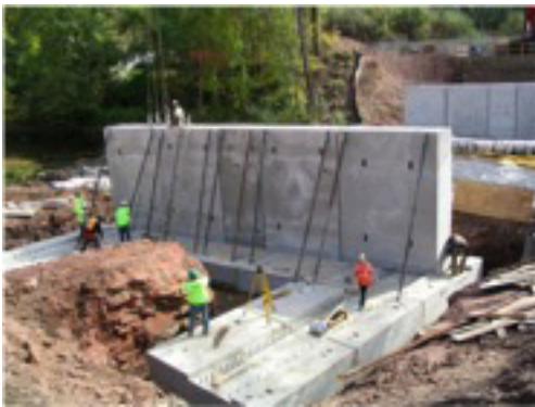
Figure 4.4.2.1-1 Vertical Joints in Abutment Wall Stem
