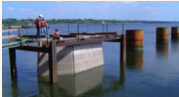
Figure 3.1.2.3-1 Precast Concrete Cofferdam.
