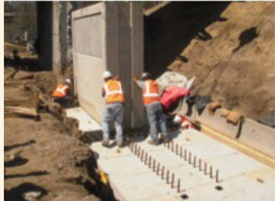
Figure 4.4.1.1 Wall Panel Installation with Mechanical Splicers
