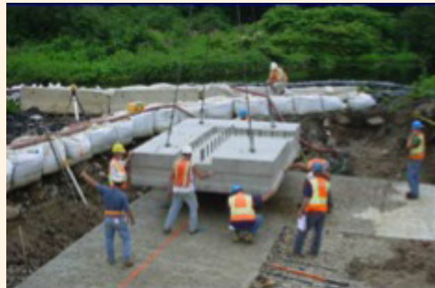
Figure 3.1.2.2-1 Placing footing segment on a sub-footing.
