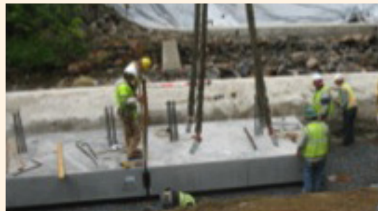
Figure 4.4.2.3-1 Precast Footings Construction
