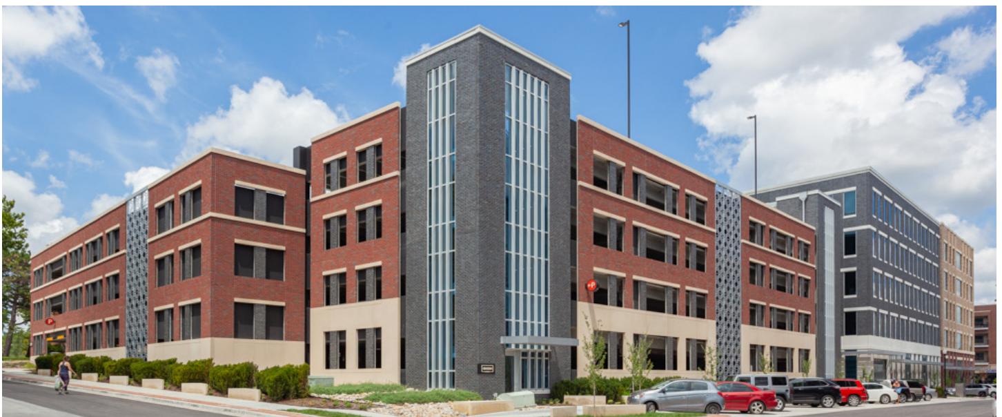
Edison District: Five-Story Mixed-Use Office Building and Parking Garage (Overland Park, KS)
