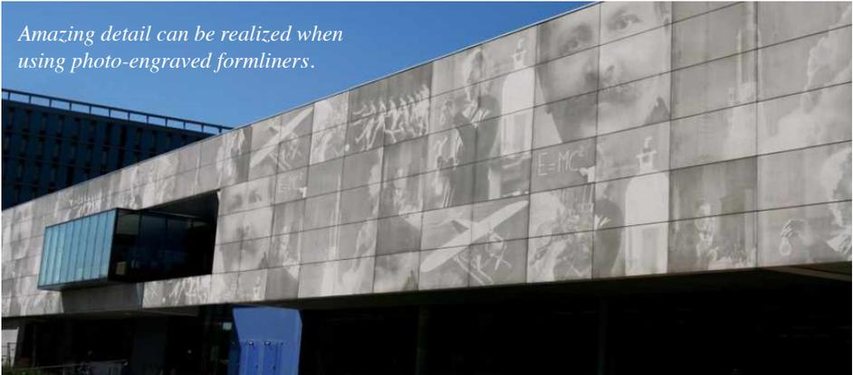
*Amazing detail can be realized when using photo-engraved formliners.*
