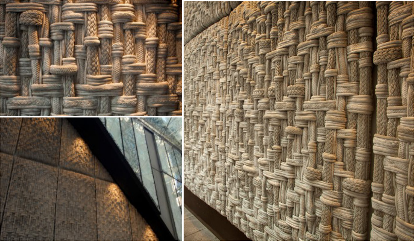
This image shows the precast concrete panel that was made from the custom rope formliner.
