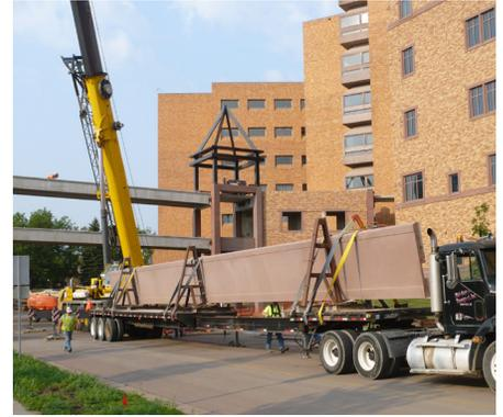
exterior finishes with a thin brick veneer cast into the panels to match the building. A complementing acid-etched finish was used on the wall panels of the skywalk's center span."
