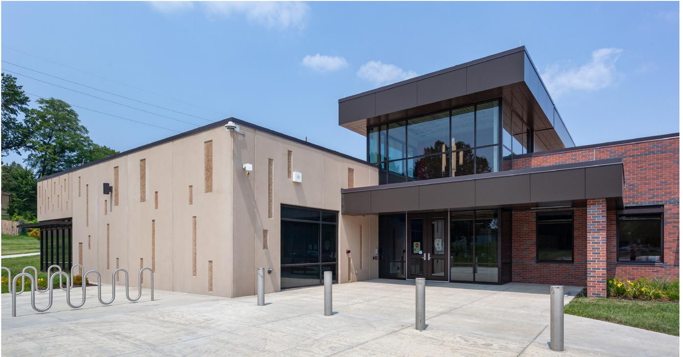
The highly ornate architectural precast concrete makes West Park Elementary School unique. The finish on this project consisted of a combination of acid etch, exposed aggregate and thin brick. There
