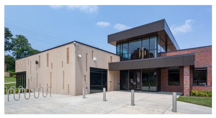
The highly ornate architectural precast concrete makes West Park Elementary School unique. The finish on this project consisted of a combination of acid etch, exposed aggregate and thin brick. There
