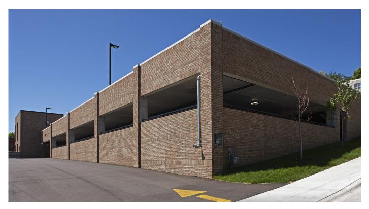
Molin Concrete worked closely with the architect and general contractor to design and build the Crosby Hotel Parking Ramp, a three-level, 124-stall parking ramp. The ramp was built to replace 35 city parking spaces that would be lost due to the planned construction of the adjacent Crosby Hotel project. Of the parking area's three levels, the first two are accessible from Mulberry Street, with the top level being accessible from Second Street.
