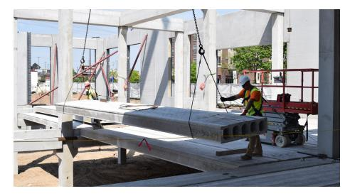
To meet the desired aesthetics, insulated and non-insulated architectural precast wall panels were used with cast-in thin brick veneer.
