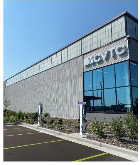
square feet of solid precast concrete wall panels and 7,800 square feet of hollow core plank. Throughout the process, Molin's project manager and field superintendent coordinated site access, crane and trucking logistics, safety, and installation plans to make sure installation was completed on budget and on schedule.
