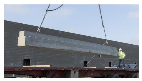
County Prestress manufactured and delivered 28,000 SF of 8-inch depth hollowcore, 32,000 SF of 12-inch depth hollowcore, and 1,666 SF of 12-inch depth solid slabs and coordinated with the contractor and erector to ensure the project was completed on time.
