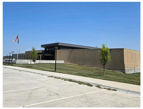
Coreslab Structures (OMAHA) Inc. produced more than 58,000 square feet of precast concrete for the project. Precast concrete was chosen for its efficiency in construction, durability, and architectural versatility. The building features buff-colored precast concrete wall panels with a light sandblast finish. A formliner was also used to enhance the visual break of large elevations. Additionally, precast concrete sign panels were integrated into the design.
