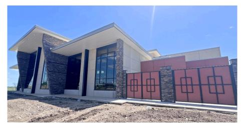
The POET Ethanol Office Expansion project highlights the intersection of architectural ambition and structural ingenuity. Designed to accommodate both aesthetic and functional needs, this expansion features bold design elements, including towering concrete fins and intricate detailing. Spanning 16,528 square feet, the project's precast concrete elements served as both structural and visual centerpieces, enabling the creation of a durable, efficient, and striking office space.
