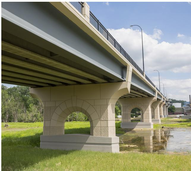
"Based on the span lengths on the Wisconsin side of the project, concrete beams were an economical solution for the superstructure," stated MnDOT Construction Manager, Terry Ward.
