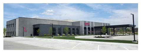
Finishes included acid etching and sandblasting on the wall panels and thin brick on the insulated sandwich panels. The colors, including an Endicott Manganese Ironspot Velour for the thin brick, were chosen to provide a sleek, modern look.
