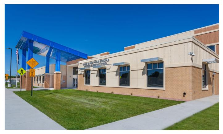
Jefferson Elementary School is one of three new elementary schools constructed by Grand Island Public Schools that incorporated the use of insulated architectural wall panels. Enterprise Precast Concrete produced the 12" thick insulated wall panels that provide an energy efficient durable exterior finish in addition to serving as the building's structural system.
