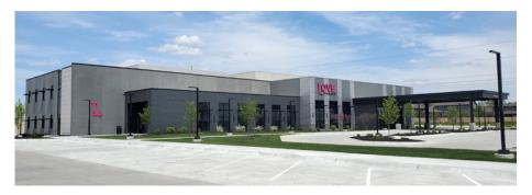
Finishes included acid etching and sandblasting on the wall panels and thin brick on the insulated sandwich panels. The colors, including an Endicott Manganese Ironspot Velour for the thin brick, were chosen to provide a sleek, modern look.
