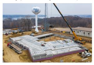
installation efficiencies. County Materials utilized its enhanced production capacity to manufacture 54,700 square feet of prestressed concrete hollowcore planks and solid slabs with short lead times.
