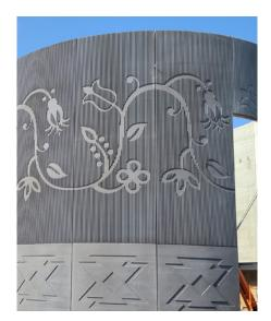
Collins Precast produced 5,490 square feet of radiused insulated precast concrete wall panels to complete a 35-foot tall, 50-foot diameter round building structure that is part of the new Lower Sioux Intergenerational Cultural Incubator. The precast concrete wall panels are 13-inches thick with four inches of embedded insulation.
