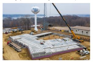
installation efficiencies. County Materials utilized its enhanced production capacity to manufacture 54,700 square feet of prestressed concrete hollowcore planks and solid slabs with short lead times.
