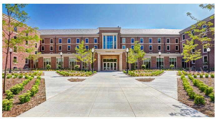
Whether adding on to an existing structure or constructing a stand-alone building that needs to match others, precast concrete can be produced precisely to match, blend with or complement those structures. An inherent benefit of utilizing precast concrete is the ability to mirror or harmonize with nearby existing structures.
