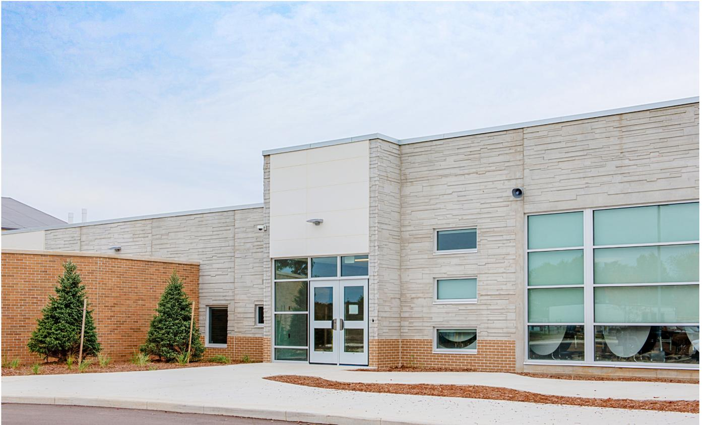
Kellogg Elementary School was originally planned as a masonry project but was converted to precast concrete due to the value it added and because it was friendlier to the project's budget. Kerkstra Precast manufactured and erected 187 insulated wall panels (35,332 square feet) and 46 six-inch solid panels (8,053 square feet) on this project. The project features thin brick as well as a wood-grain form liner finish.
