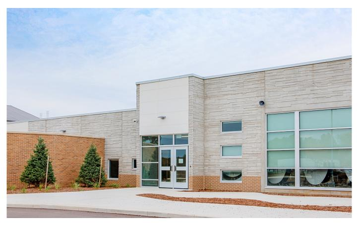
Kellogg Elementary School was originally planned as a masonry project but was converted to precast concrete due to the value it added and because it was friendlier to the project's budget. Kerkstra Precast manufactured and erected 187 insulated wall panels (35,332 square feet) and 46 sixinch solid panels (8,053 square feet) on this project. The project features thin brick as well as a wood-grain form liner finish.
