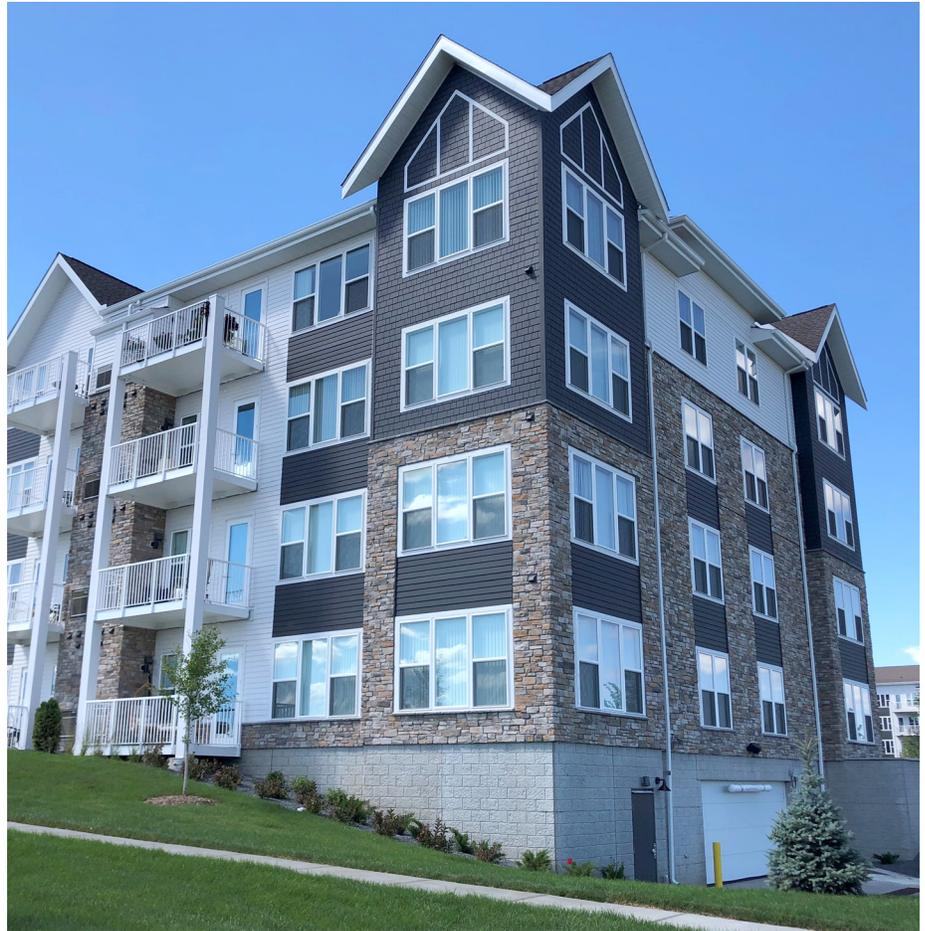
colored mix. Molin contributed 54,887 square feet of hollow core, 1,772 lineal feet of prestressed beams, 645 lineal feet of precast columns, 1,502 square feet of solid slabs, and 31,168 square feet of architectural precast wall panels.
