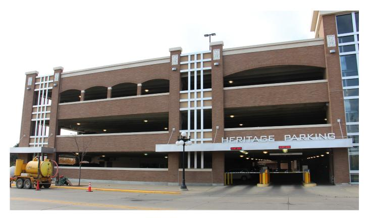
Precast concrete is the perfect solution for parking structures because it arrives at the site ready for installation and does not require protection from rain, sun, snow, wind, or extreme temperatures. This saves time and money and reduces the potential for change orders due to winter conditions.
