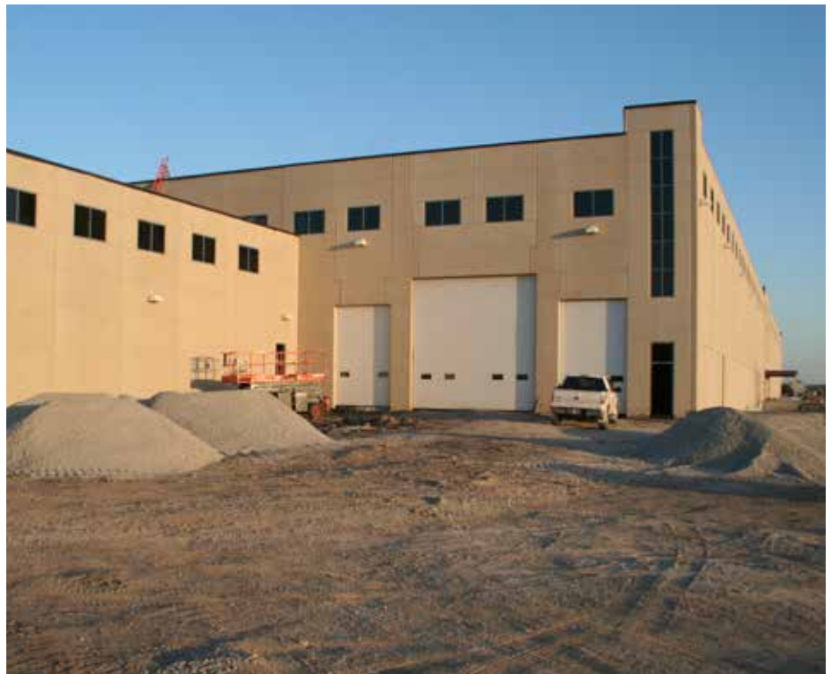
Owner: Lincoln Airport Authority • Architect/Engineer: Davis Design • Contractor: NGC Group, Inc. • Location: Lincoln, NE
