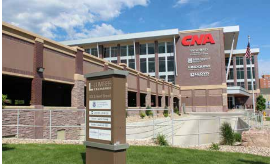
Owner: Lloyd Companies • Architect: Perspective, Inc. • Structural Engineer: BKBM Engineers • Contractor: Lloyd Companie • Location: Sioux Falls, SD
