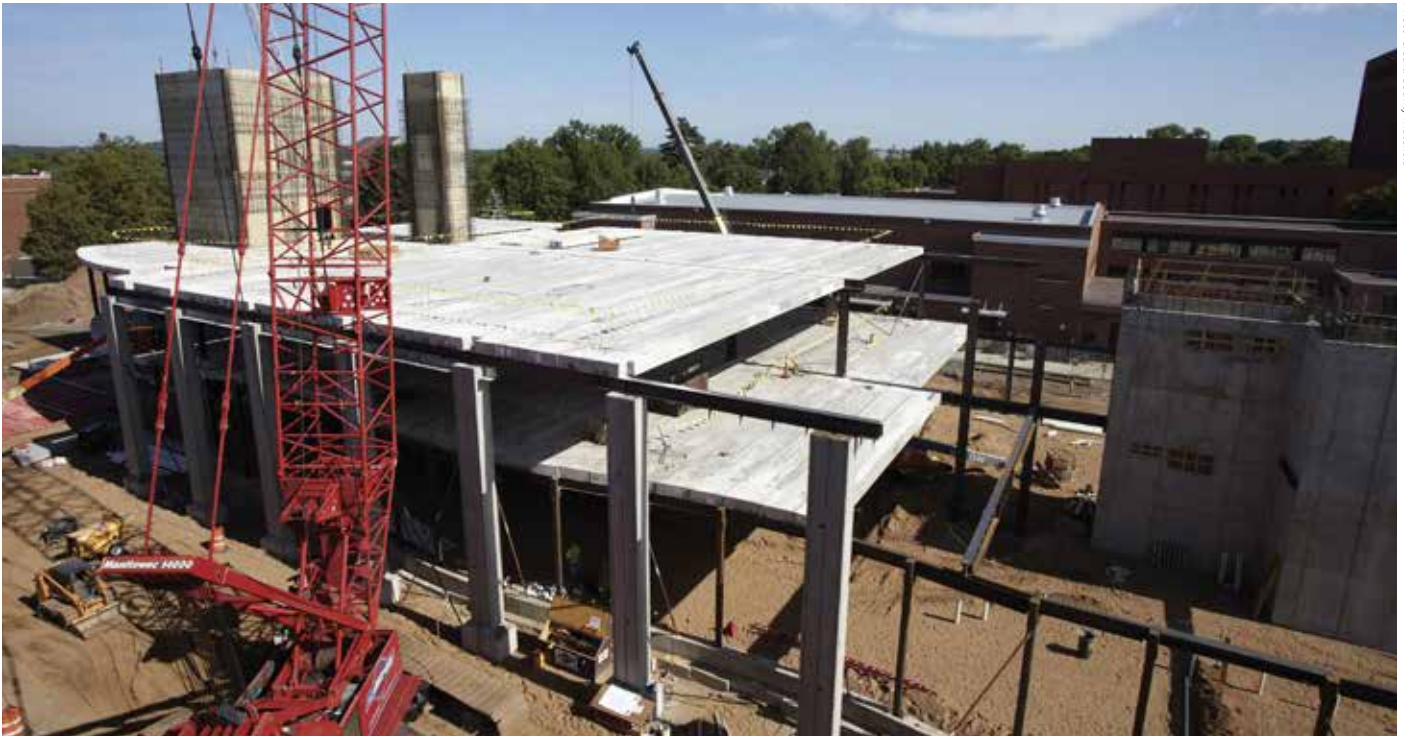
Photo Credit: County Materials
