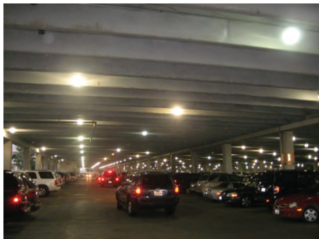
Figure 1-11. Typical interior view of precast concrete structure showing long, clear spans
