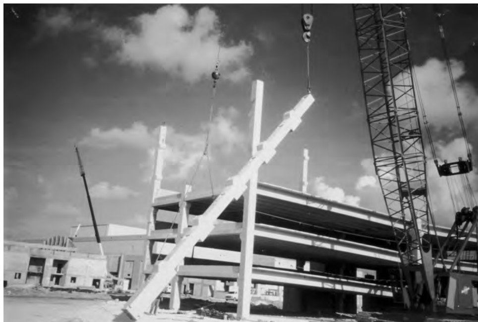
Figure 8-3 Rotating a column into position.
