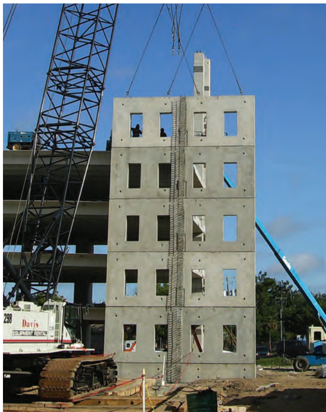
Figure 8-6 Story-height wall panels “Stacked.”
