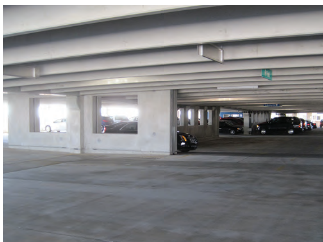
Figure 1-12. Typical view of openings in shear walls
