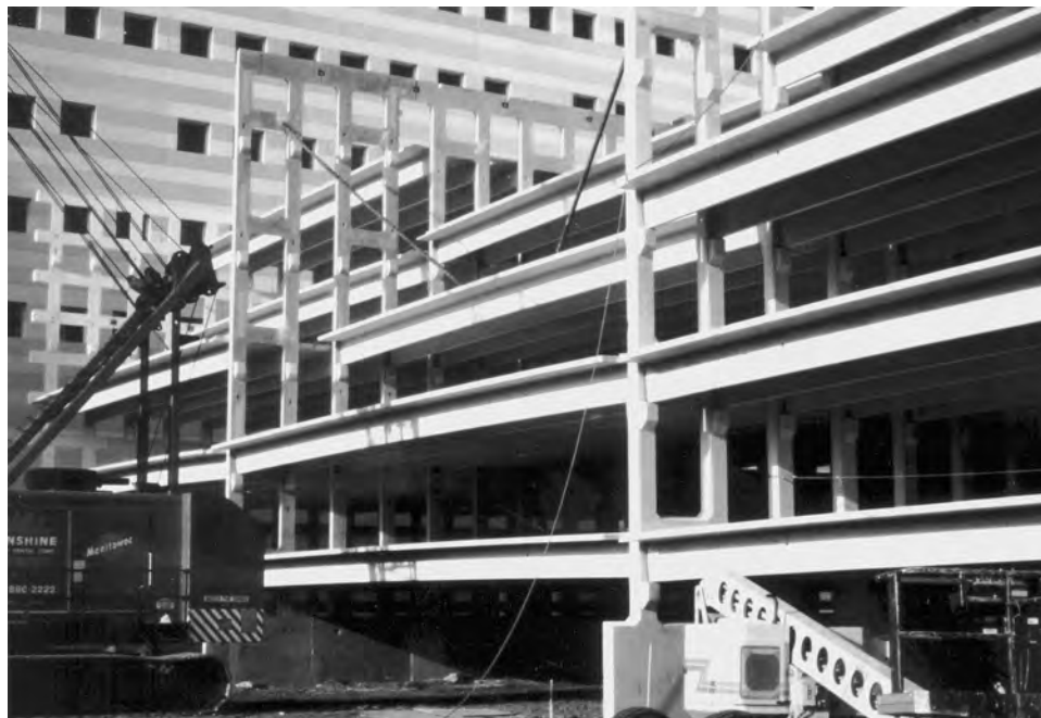
Figure 8-7 Braced litewalls during erection.
