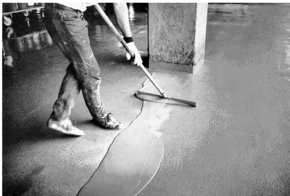
Figure 3-6 Application of Deck Membrane
