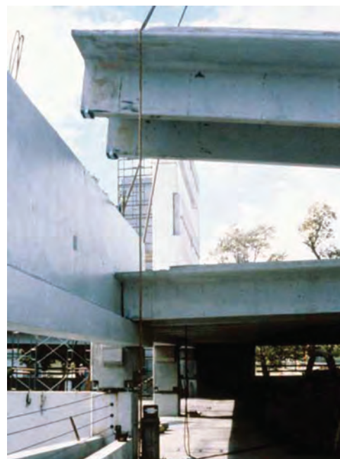
Figure 8-5 L-shaped spandrel being loaded with double tees.
