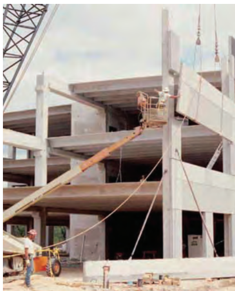
Figure 8-4 Spandrels being erected into pocketed columns.
