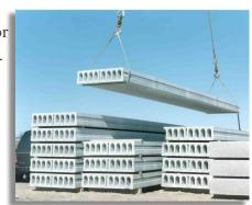
Hollowcore products typically are cast in 300- to 800 foot long prestressed casting beds with at least one system mak-
