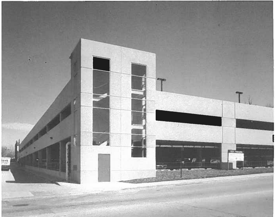
The Naperville Municipal Parking Structure, Naperville, Ill., went from approval to completion in just over five months — proof of the fast-track construction schedules that can be met with Precast/prestressed concrete.
