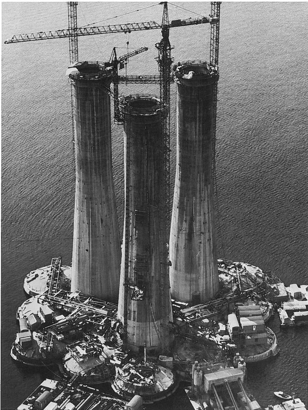
The cyclic dynamic loading of storm waves on towers such as these of Condeep, requires design to prevent fatigue.
