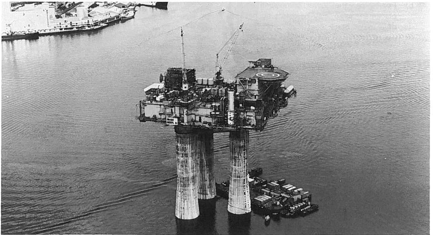
Condeep Beryl A: This huge concrete structure, largely submerged at this stage, has just "picked up" the 12,000 ton deck structure.
