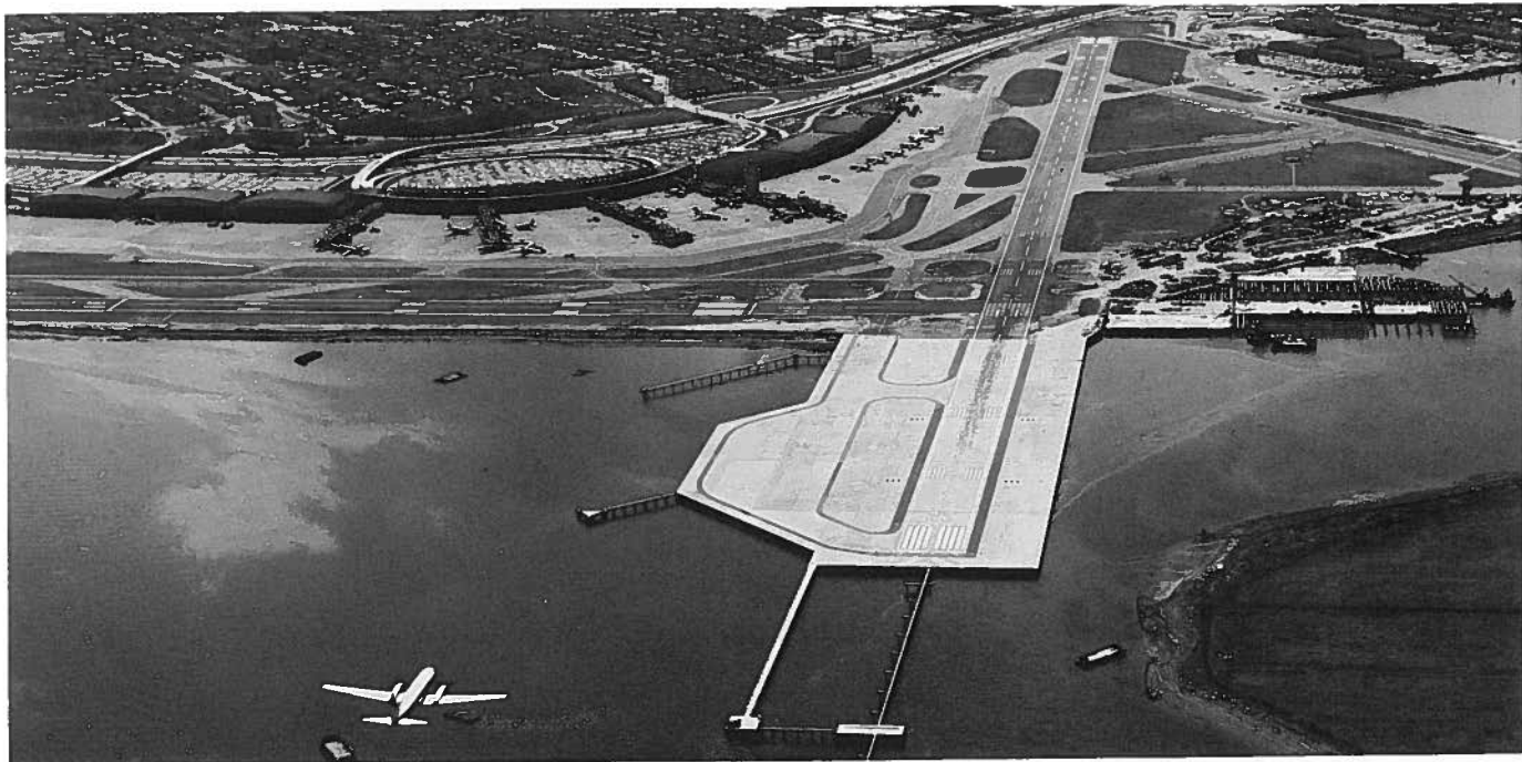
Over-water extension for La Guardia Airport was constructed of precast pretensioned segments, connected by post-tensioning and cast-in-place concrete for monolithic behavior.
