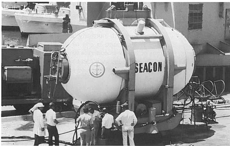
56" diameter thin-wall concrete spheres which have been subsequently installed at sea in depths to 3000 feet.
