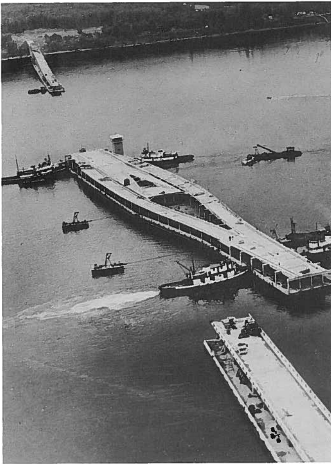
Hood Canal Bridge pontoons were assembled afloat into rigid structures by post-tensioning and epoxy.
