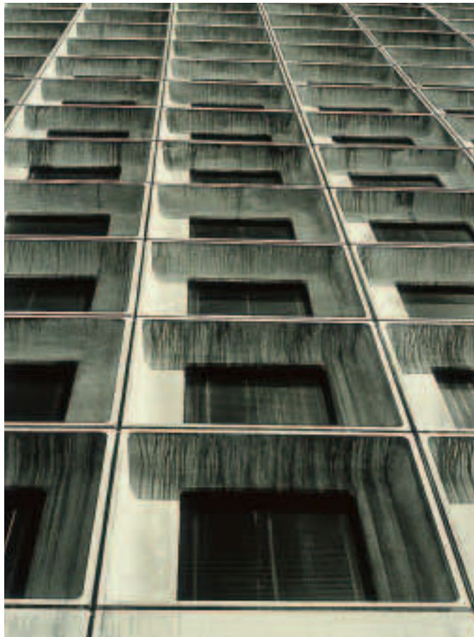
Fig. 32. Aesthetics can be destroyed by lack of detailing for weather.
