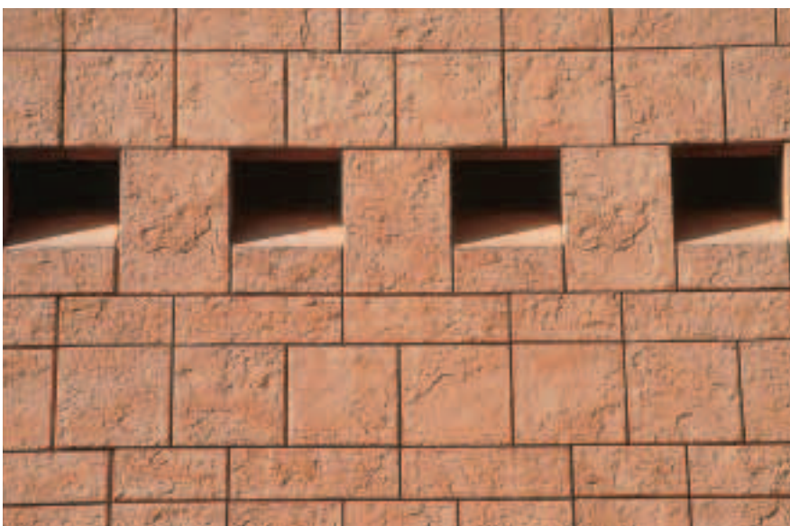
Fig. 23. Form liners were used to achieve stone texture of panels.
