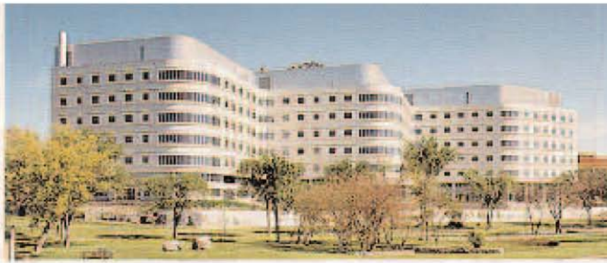
Fig. 21a. Saskatoon City Hospital walls are precast concrete sandwich panels incorporating insulation and a rain screen, with ceramic tile on the exterior. Architect: City Hospital Architects Group, Inc., Saskatoon, Saskatchewan, Canada, a Joint Venture of Folsstad & Friggstad Architects, Billington Poon Associates Ltd. and Arthur Erickson Architects.
