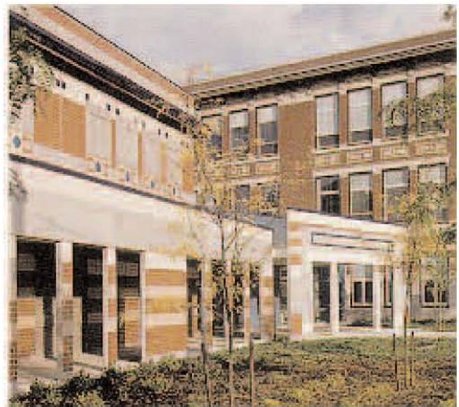
Fig. 22. The Ravenna Eckstein Community Center in Seattle, Washington uses precast concrete panels articulated with reveals and recesses varying from 3/4 to 1 1/4 in. (19 to 35 mm) to reflect the adjacent 1911 school's proportions. Ceramic tile was then selectively field-laid on the concrete to reference the school's brick and terra cotta banding and details. Architect: ARC Architects, Seattle, Washington.
