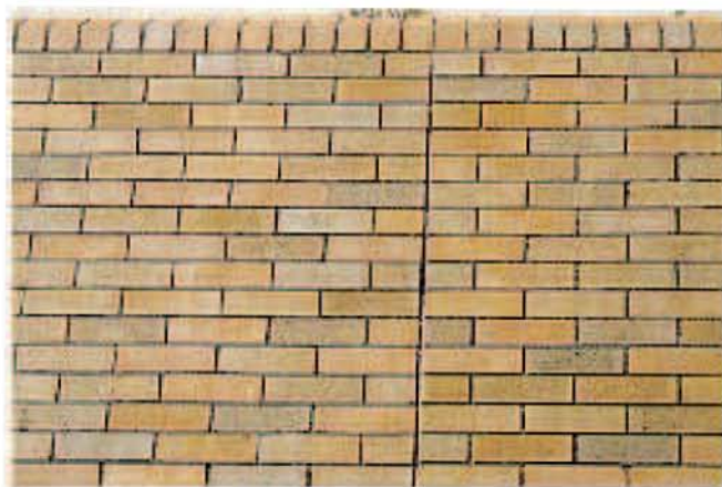
Fig. 3. Brick patterns must be continuous through adjacent panels.
