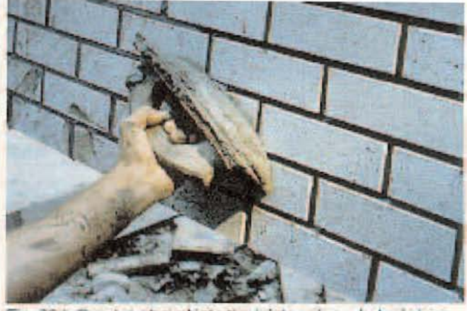
Fig. 20d. Grout is placed into the joints using a baker's bag or large caulking gun. Excess grout is struck from the brick surface using a rubber-faced float. The float is worked at 45 degrees to the surface.
