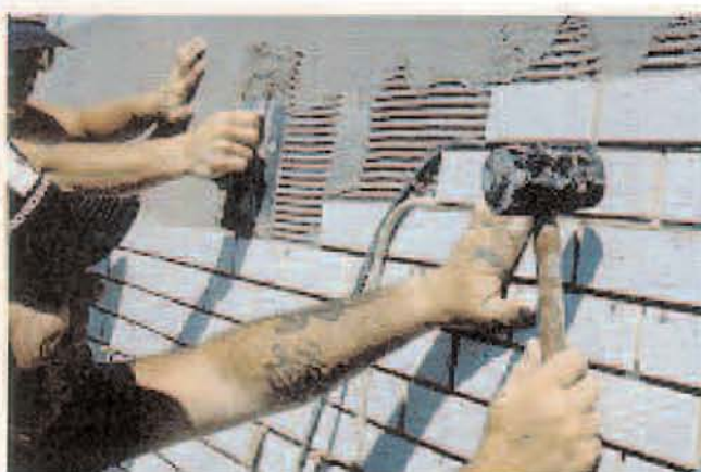
Fig. 20c. The bricks are tapped into the mortar using a rubber mallet. Level and alignment are also checked at this point.
