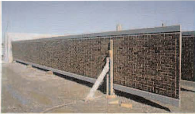
Fig. 17. A vertical easel was an effective restraint for 65 ft (19.8 m) long prestressed concrete panels during stockpiling.
