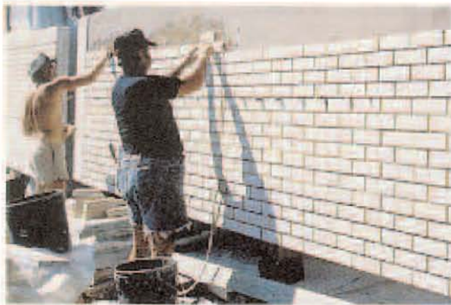
Fig. 20b. A second coat of mortar is applied to the panel surface using a notched trowel. The glazed brick is then applied to the panel surface.
