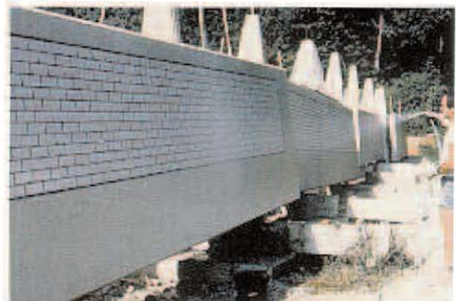
Fig. 20f. After the grout has cured, the panel is cleaned using stiff brushes and then rinsed with low-pressure water.
