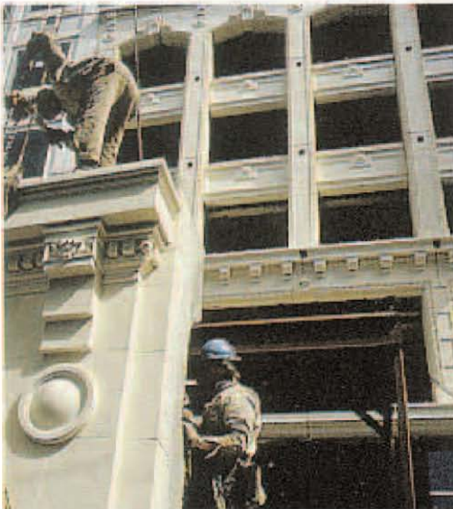
Fig. 10. Built in 1906, the six-story 88 Kearney St. is considered one of San Francisco's architectural landmarks. For that reason, it was decided that the building's terra cotta facade would be preserved on an otherwise all-new structure of slightly taller height. The terra cotta was taken off the building, piece by piece, and the pieces were identified for subsequent reassembly on new precast concrete panels. Architect: Skidmore, Owings and Merrill, San Francisco, California.
