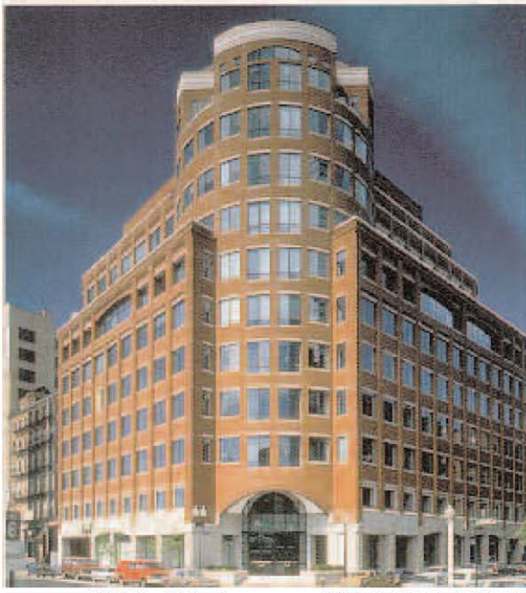
Fig. 6. Brick-clad precast concrete panels were used to speed up the construction time required for the 10-story office building at 745 Atlantic Avenue, Boston, Massachusetts. Corbeled brick, concrete sills and lintels, and recessed windows with arches continue the architectural vocabulary of the surrounding older buildings. Architect: The Stubbins Associates, Inc., Cambridge, Massachusetts.
