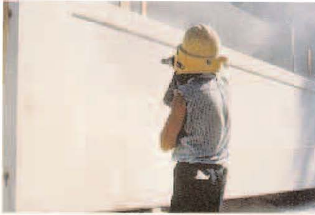
Fig. 20a. The surface of the panel is lightly sandblasted prior to parging with a skim coat of latex-portland cement mortar.
