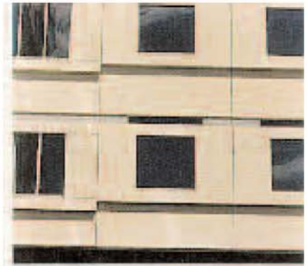
Fig. 21b. The paper-faced 2 in. (50 mm) square tiles on a 1 ft (0.3 m) square sheet were applied in the plant using latex-portland cement mortar and easily adapted to the complex wall profiles.
