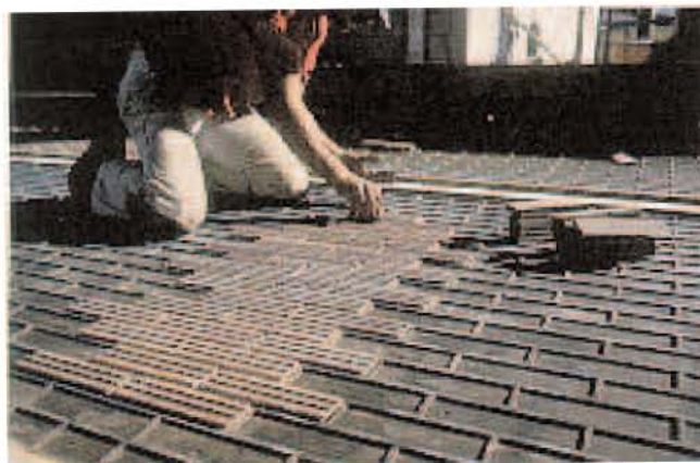
Fig. 13. Thin brick being placed in elastomeric form liner.
