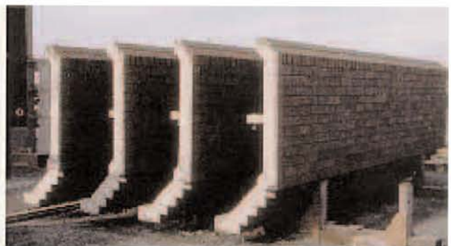
Fig. 16. Support framing is kept away from brick edges to prevent spalling.
