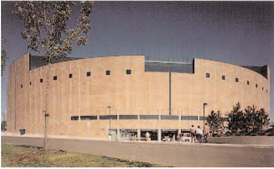
Fig. 7a. The Palace of Auburn Hills, Auburn Hills, Michigan, is clad with 9 in. (225 mm) thick curved precast concrete panels cast with a contrasting basketweave pattern of 8 in. (200 mm) square, 2 in. (50 mm) thick brick units and a rectilinear grid of blue-green glazed brick. Architect: Rossetti Associates, Detroit, Michigan.
