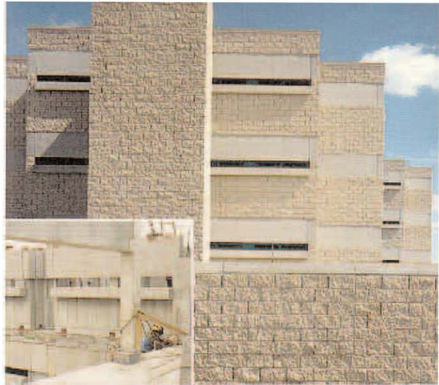
Fig. 25. Panels for the Oakland County Jail Addition in Pontiac, Michigan, were delivered to the site complete with slots for dovetail anchors to support split face block. Architect: NSA-HDR — A Joint Venture, Southfield, Michigan.
