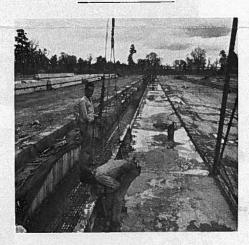
Capitol Concrete Co., Jacksonville, Florida, is currently producing prestressed concrete piling 20" square at the rate of 400 linear feet per day for State Road Department bridge over Trout River at Jacksonville's north city limits. The 732-ft.-long bridge will require a total of 7,800 lin. ft. of piling varying in lengths from 59 to 66 ft. Duval Engineering & Construction Co. holds the \$483,-514 contract.
