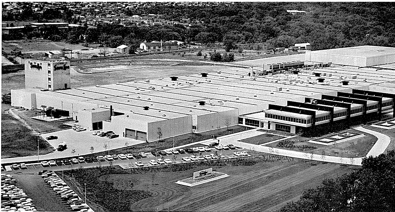
Architect-Engineer: A. Epstein & Sons, Inc.; Prestressed Concrete: Material Service
