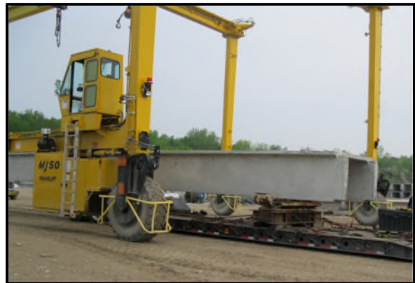
Typical loading arrangements for Double Tee product.
