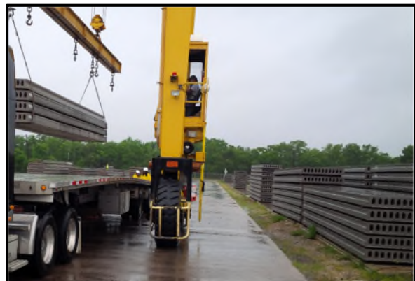
Typical loading arrangements for wall panel and hollow core floor product.
