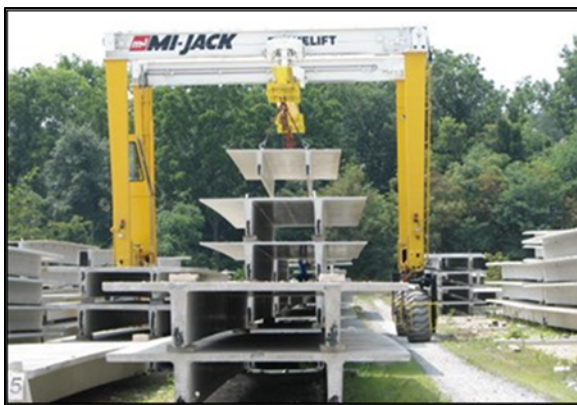
Typical stacking arrangements for double-tee product in storage yard
