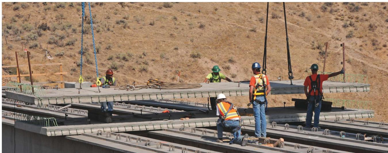
Full-depth deck panel being installed using a four-point pick. Photo: Precast/Prestressed Concrete Institute.
