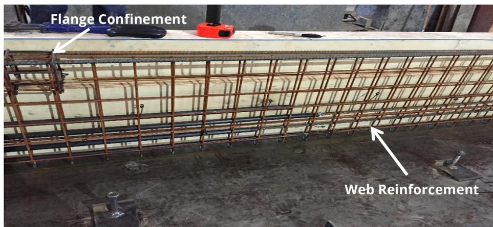
**Figure 4. WWF Reinforcement**
