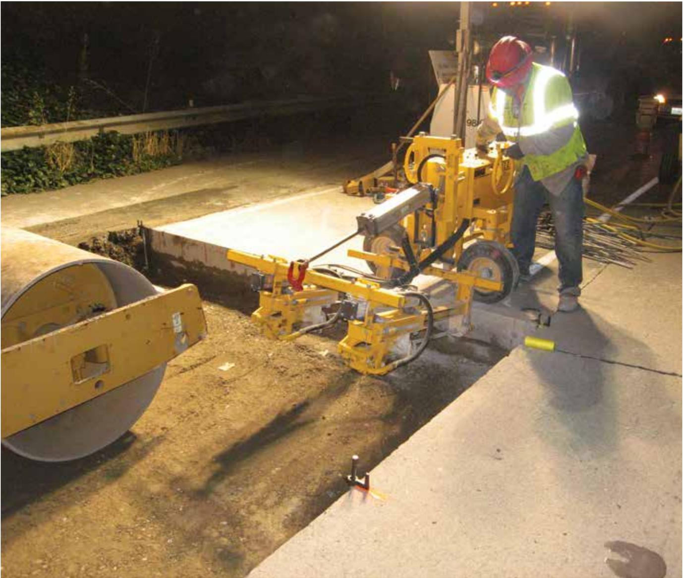
**Figure 5.** Drilling dowel slots.
