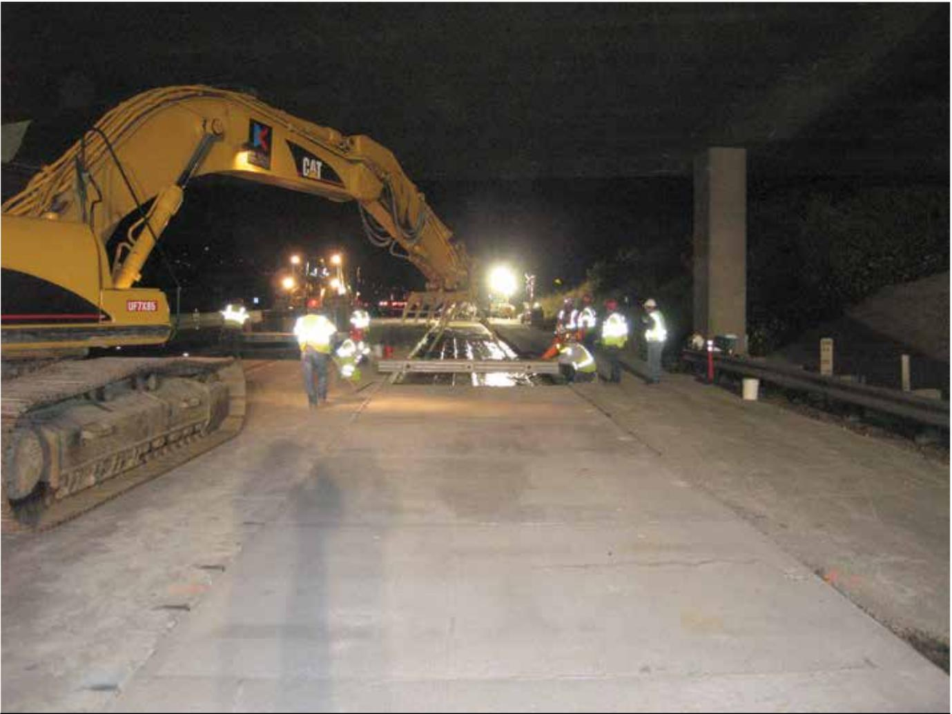
**Figure 10.** Precast, posttensioned concrete pavement installation under a structure (17 ft [5.2 m] clearance).
