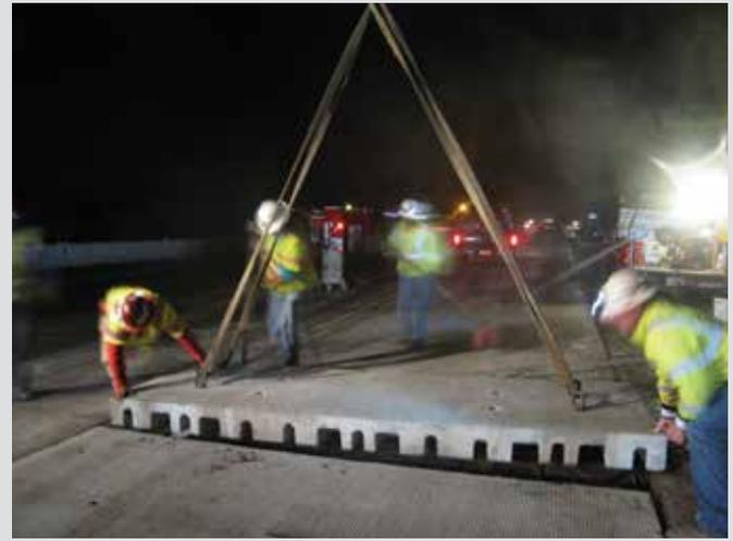
**Figure 8.** Final posttensioning and placement of temporary drop-in panel.
