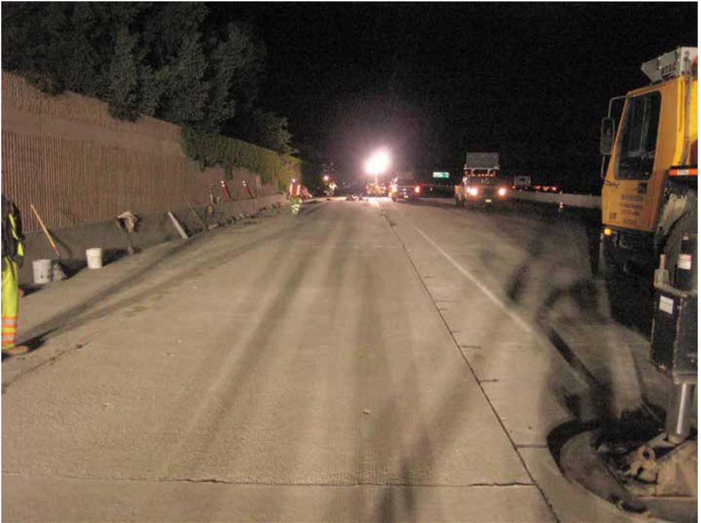
**Figure 9.** Completed precast, posttensioned concrete pavement.
