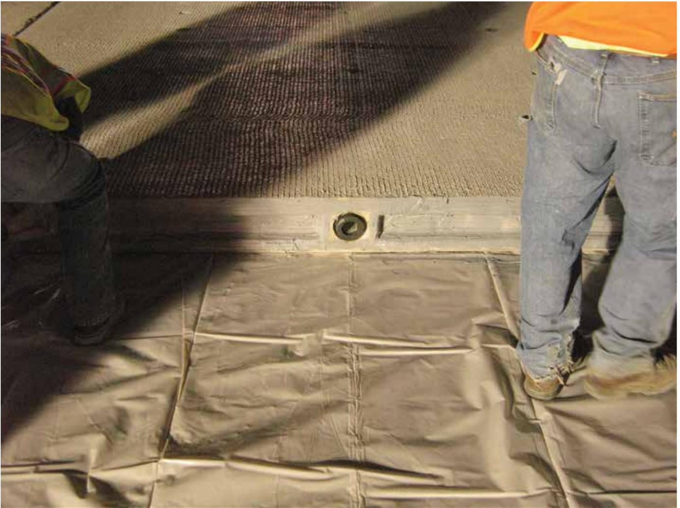
**Figure 2.** Keyway and 2 in. (50 mm) diameter posttensioning ducts between precast, posttensioned concrete pavement panels.
