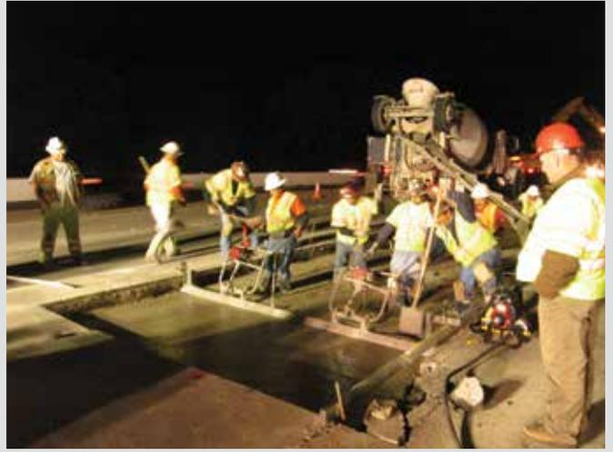
**Figure 6.** Placing and grading lean concrete base.
