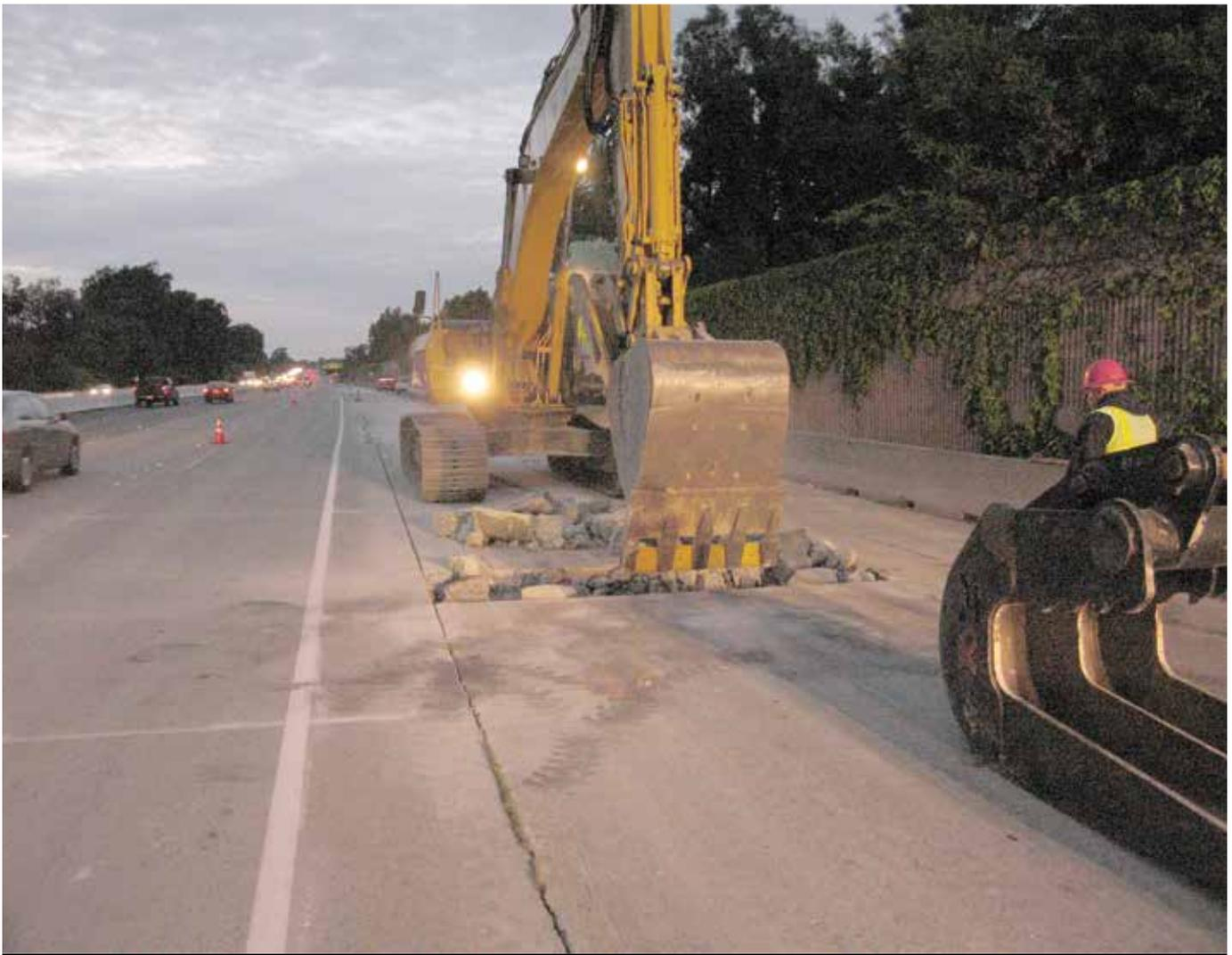
**Figure 4.** Demolition of distressed pavement and underlying base.
